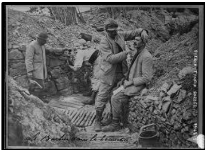
Soldiers in the Trenches
